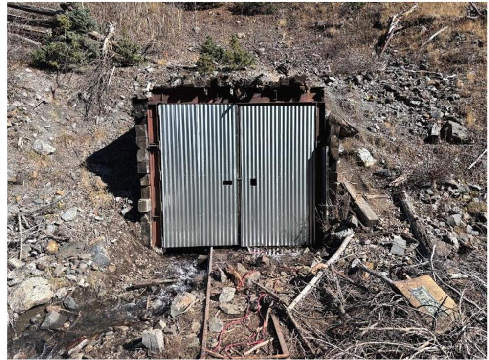
Installed metal deck panels in the first two steel sets underground, new door with better lock shrounding and new door cover.
