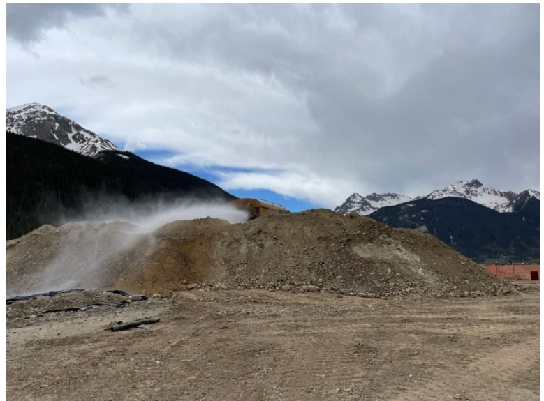
Water truck sprays down a pile of material for dust suppression.
