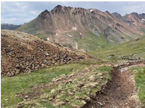
Drainage swale at the Vermillion Mine
