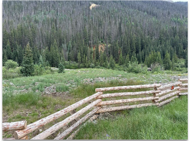
Vegetated soil cover at tresspass Campground 4 constructed as an interim action
