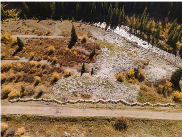
Aerial view of fencing installed at Campground 4
