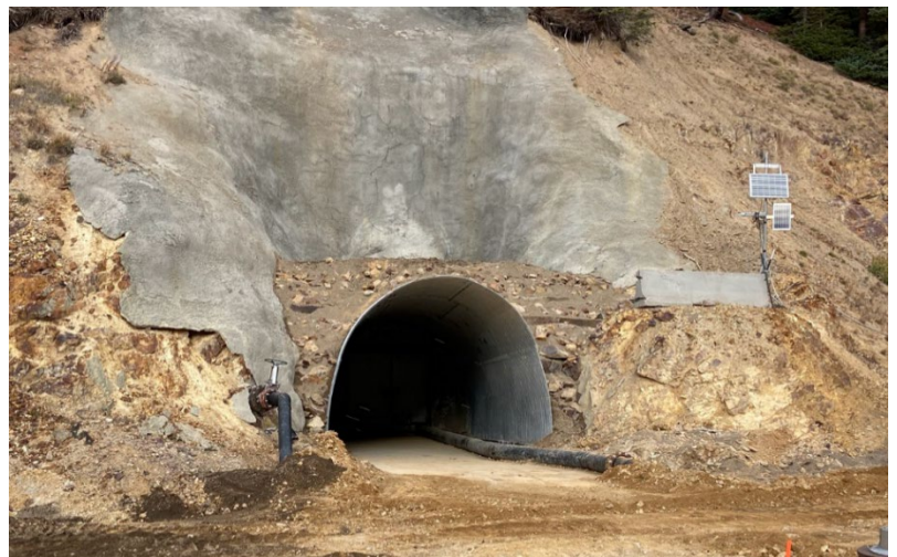
Completed portal extension at Gold King Mine
