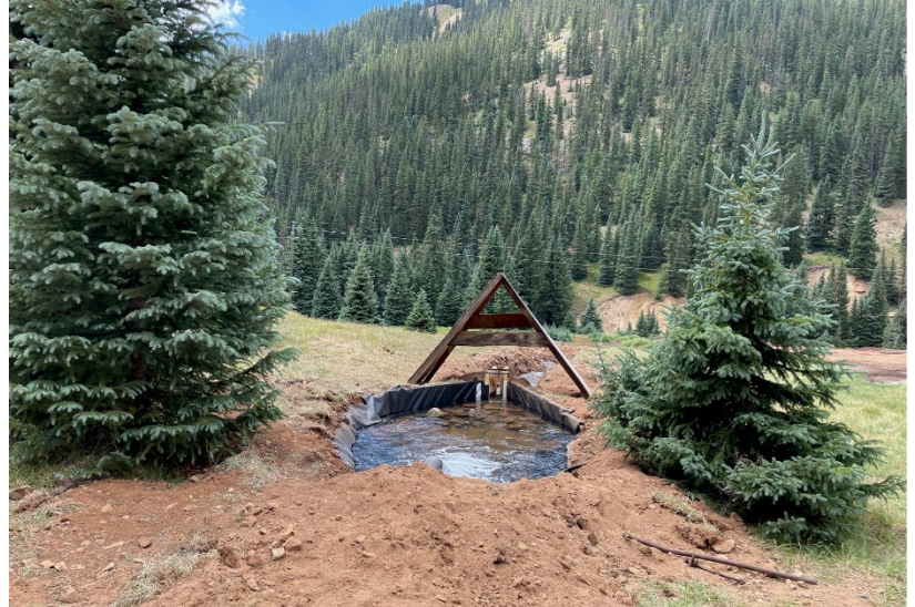
Adjusted drainage at Red & Bonita
