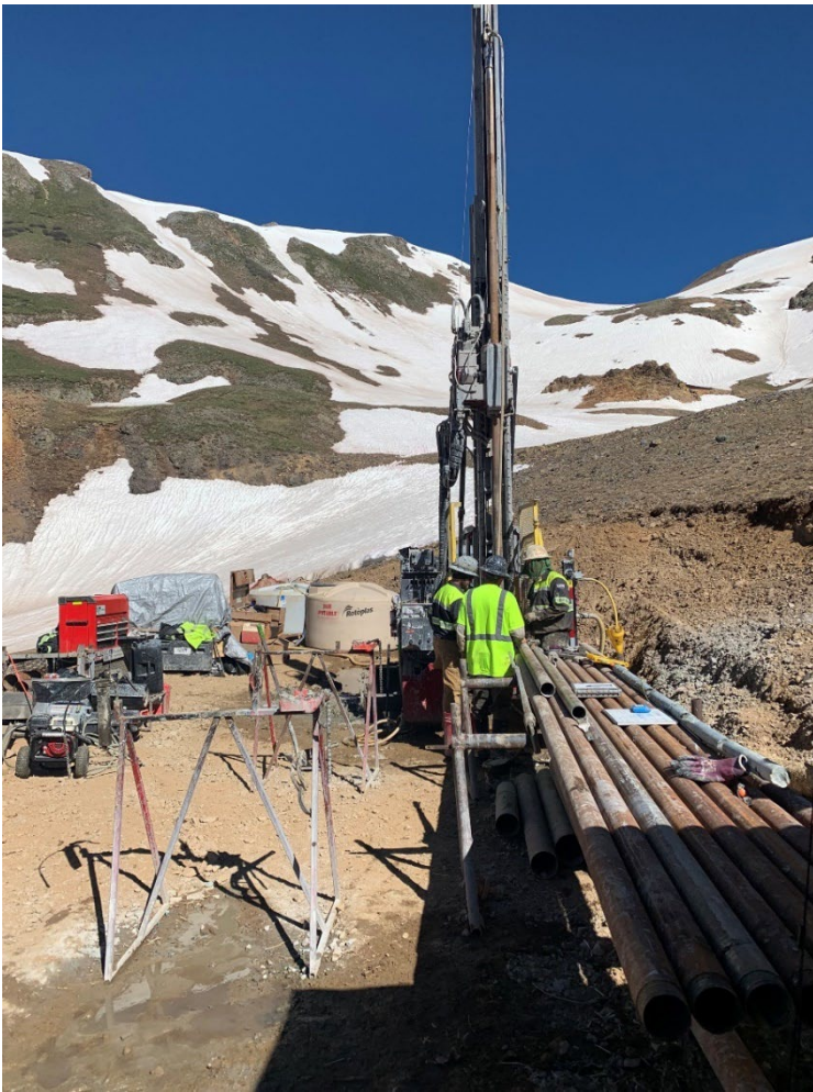
Drilling Equipment at Lake Emma in early July
