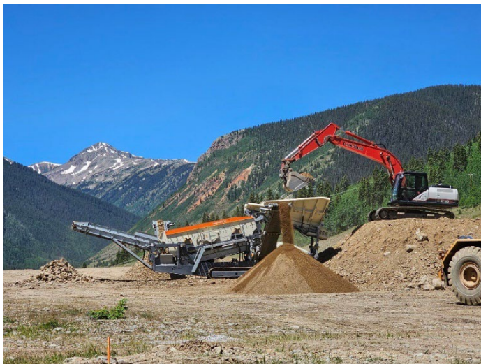
Screening material at the Bonita Peak Repository site
