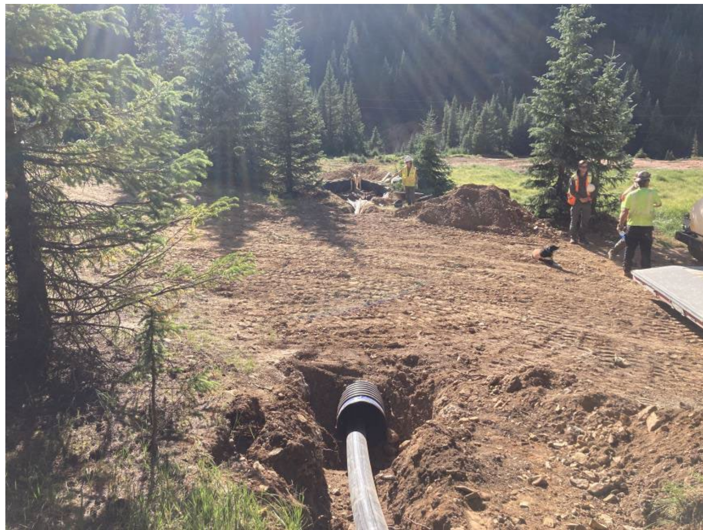
Red & Bonita Mine Drainage Relocation
