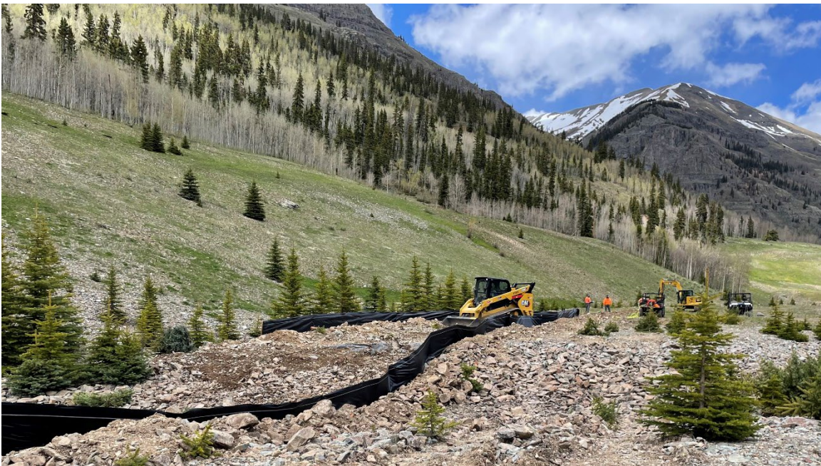
Repository construction on Tailings Impoundment 4 Photo: EPA
