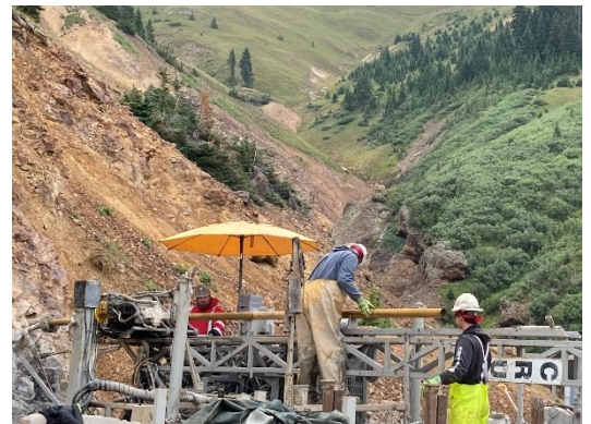
Gold King Mine borehole work
