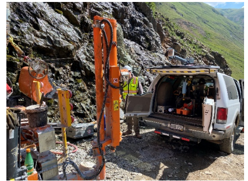
Terry Tunnel drilling work
