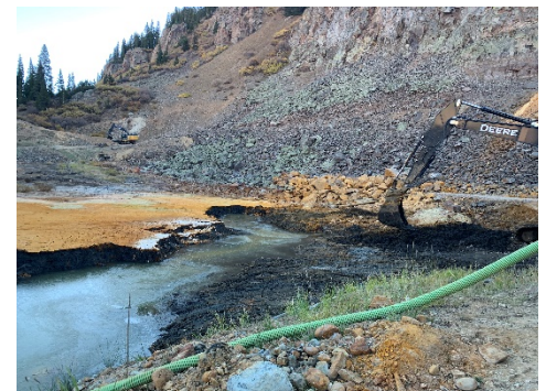
Figure 2: Kohler Tunnel sediment removal
