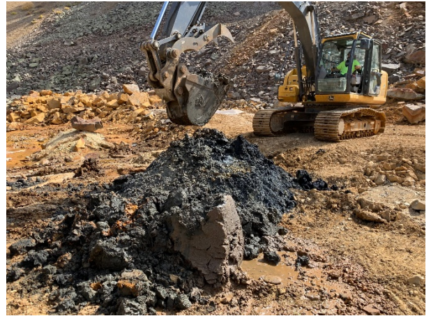
Contractors begin the sludge removal process at the Kohler Mine.
